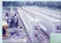
RC post tensioned girders
