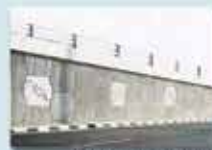
Reinforced earth wall
